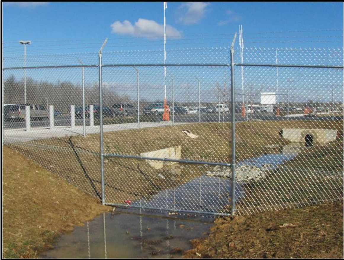
Figure 2-15- Chain Link Fence over Ditch
